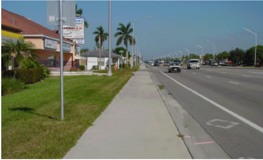
US 41 lacks a landscape buffer between road and sidewalk. High traffic speeds deter pedestrianism. Businesses are set back from US 41, making it difficult to notice businesses.
