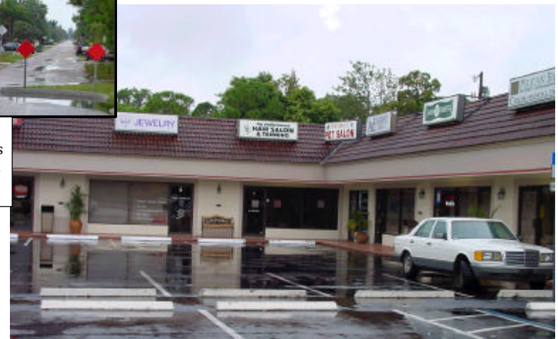
Businesses in Sunset Plaza receive less patronage due to a road block preventing through traffic down 108th Street to US 41.
