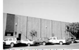
This building with its minimal detailing and windows does not respond to the sidewalk-level or human scale.
