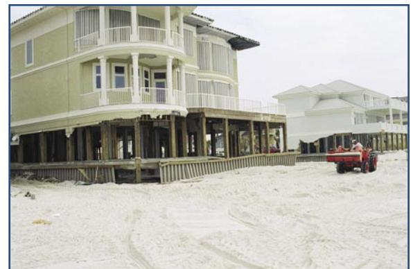
Breakaway walls that failed under the flood forces of Hurricane Ivan.
