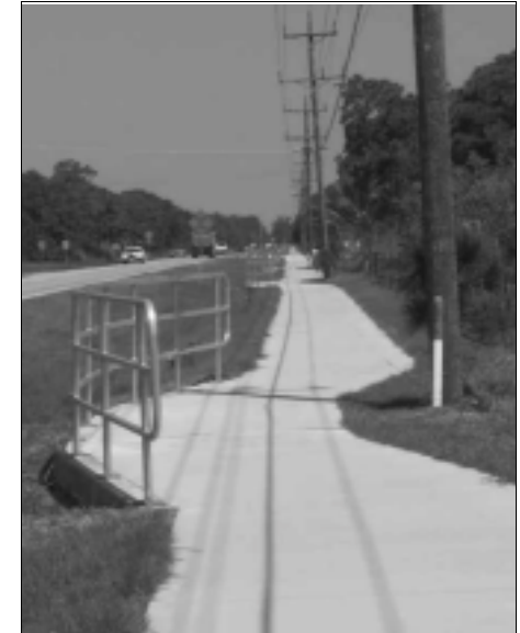
The result of moving the path rather than moving the poles
