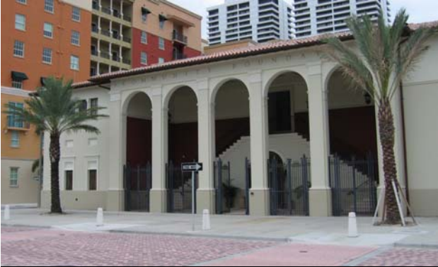
TYPE III BUILDING: Community Foundation
