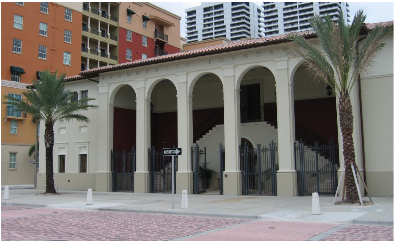
TYPE III BUILDING: Community Foundation
