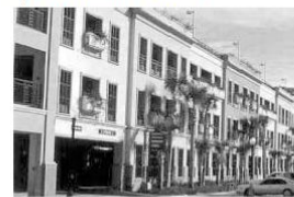
Variations or “articulation” of a building facade help in creating human scale, even on the outside of a parking garage as shown above.
