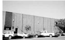
This building with its minimal detailing and windows does not respond to the sidewalk-level or human scale.
