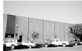
This building with its minimal detailing and windows does not respond to the sidewalk-level or human scale.
