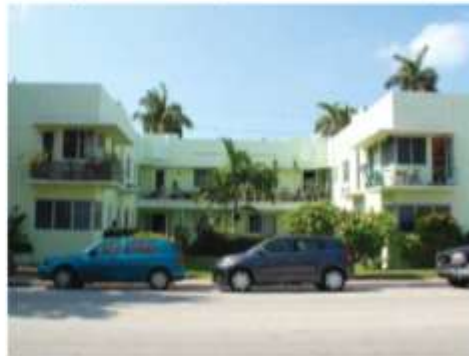
Courtyard Building Character Examples
