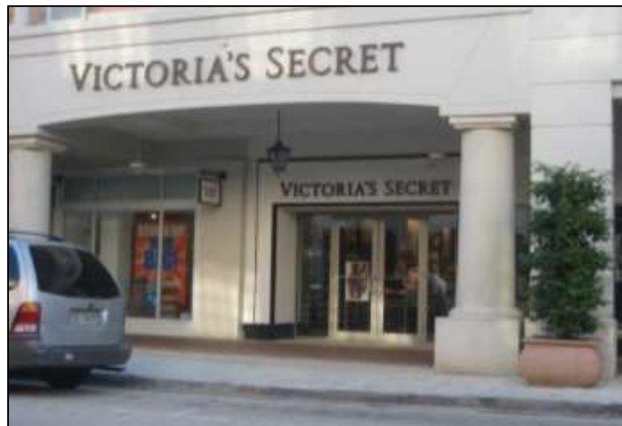
Arcade/ Colonnade Signage Examples
