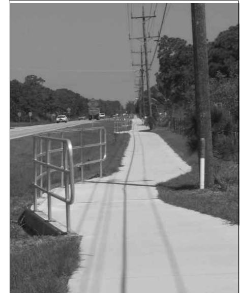
Moving the path rather than the poles
