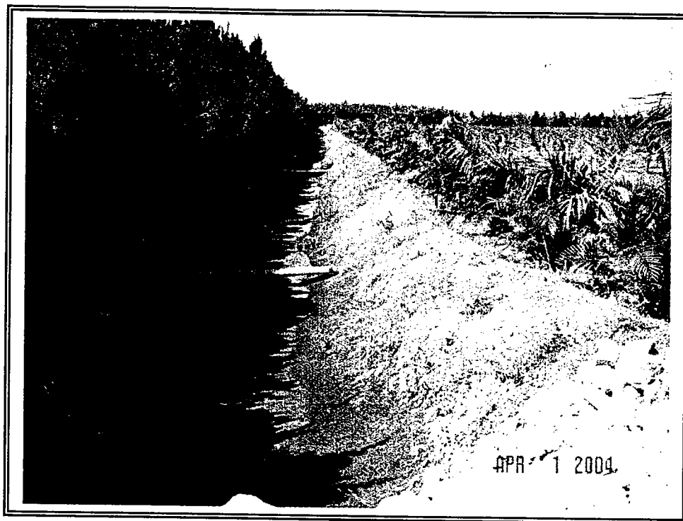
Photo No. 7: Photograph of perimeter ditch at active palm grove facility.
