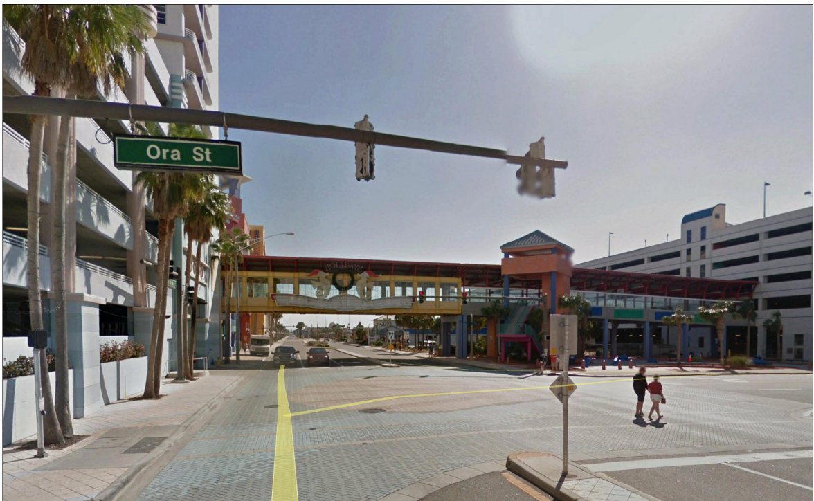
Pedestrian Bridge at Ocean Walk, Daytona Beach
