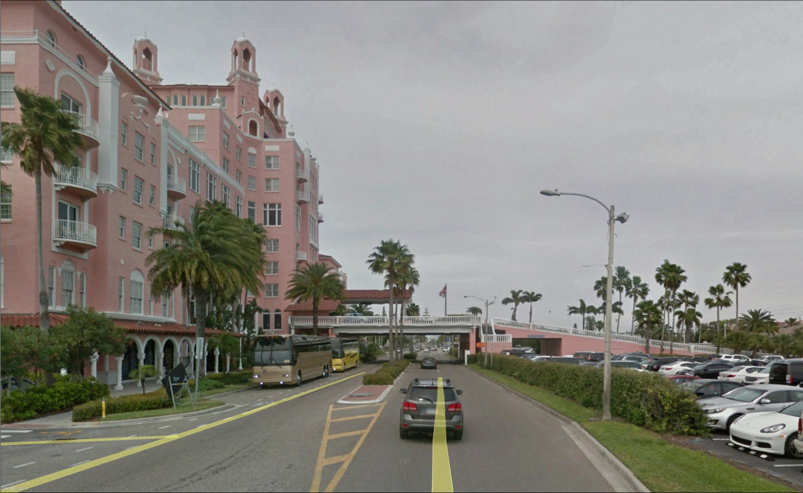
Pedestrian Bridge at Don Cesar, St. Petersburg Beach
