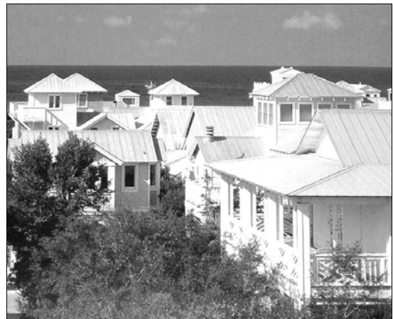
Roofed towers, Figure 34-1-b
