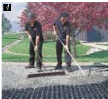
Fill rings with clean gravel.
