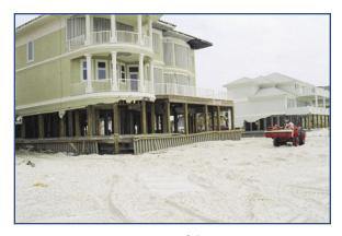
Breakaway walls that failed under the flood forces of Hurricane Ivan.
