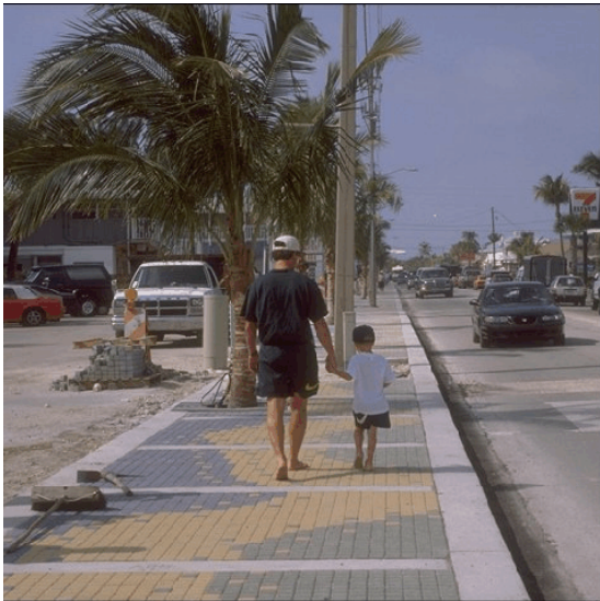
Figure 13 , CRA sidewalks during construction
