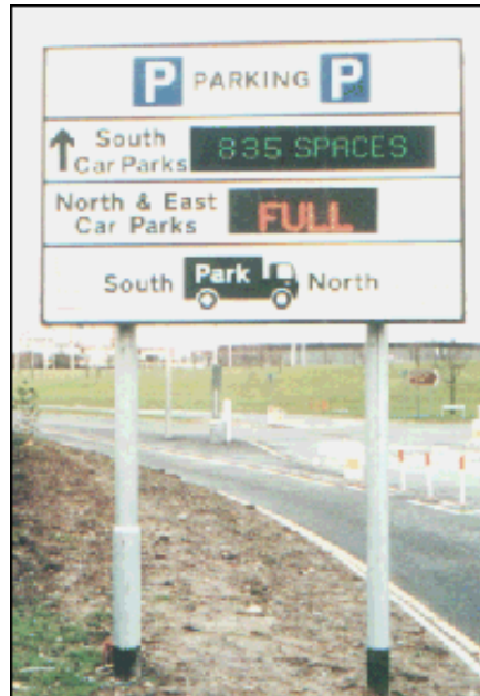
Figure 21. Variable message sign for parking management
