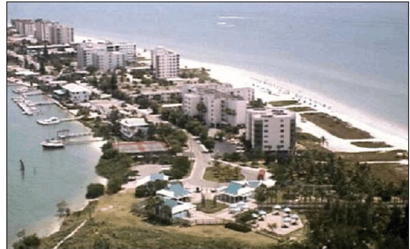
Figure 1 , Aerial view from the north end of Estero Island, with Bowditch Point Regional Park in the foreground (photo courtesy Mohsen Salehi)
