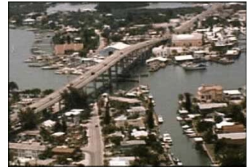
Figure 17 , Sky bridge over Matanzas Pass (photo courtesy Mohsen Salehi)
