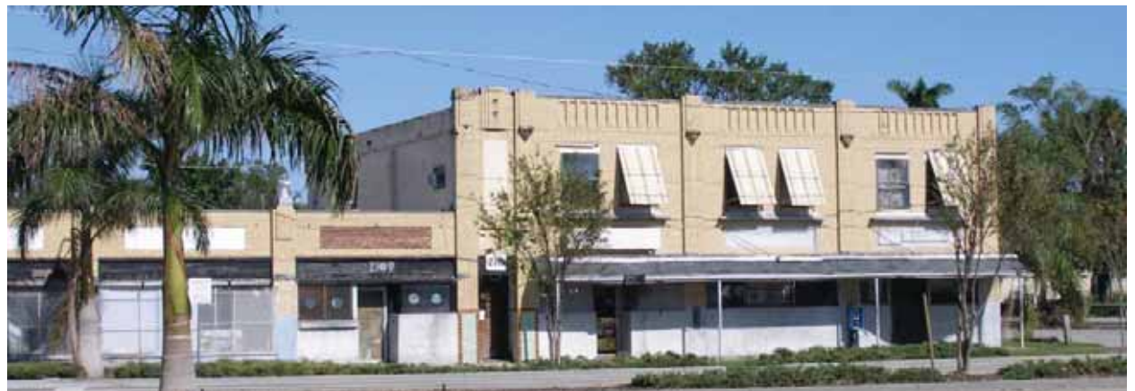
Buildings in Dunbar, such as McCollum Hall, are waiting for reinvestment.
