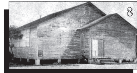
THE 1942 ADDITION TO THE WILLIAMS ACADEMY 1936 HENDERSON AVENUE - CLEMENTE PARK
