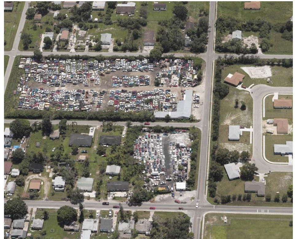
Looking south at existing junkyards at Henderson Av. and Edison Av.
