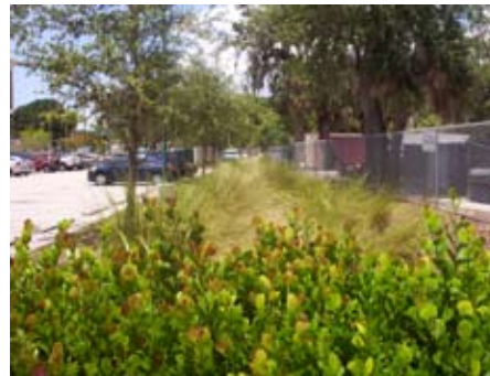
Figure 6.18: Drainage swale planted with natives
