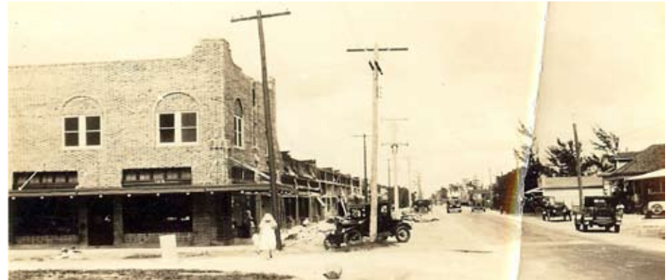
Figure 1.33: Starnes Building after 1926 hurricane. 17
