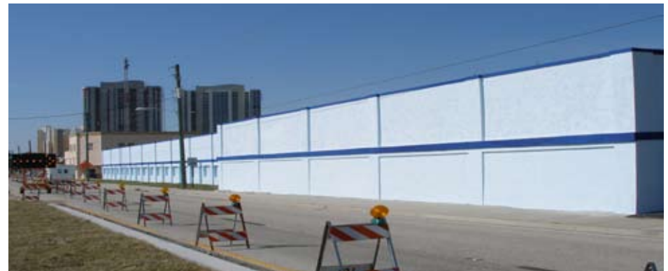
Figure 1.34: Starnes Building in 2007, after prior road widenings but during median installation 18
