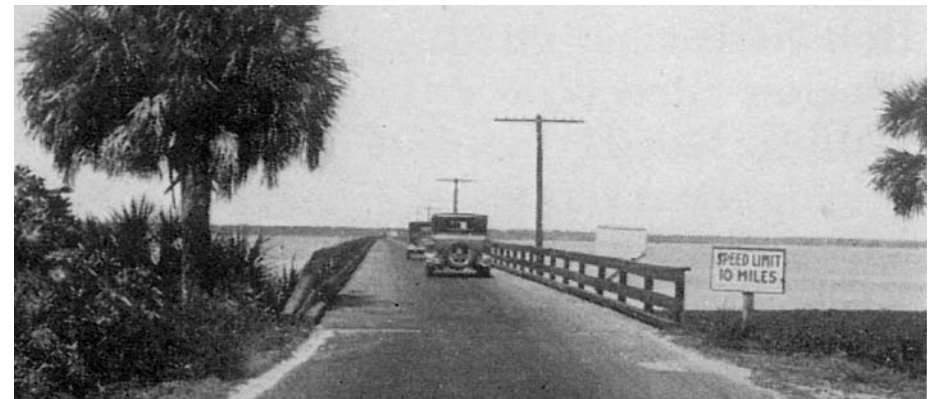
Figure 1.25: "Caloosahatchee River highway bridge" in 1926 9
