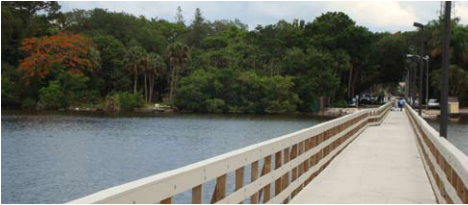
Figure 1.5: The Tarpon Street Pier provides public access to the Caloosahatchee River.
