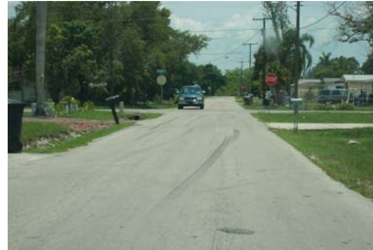
Figure 5.16: Typical Street on South Side of Palm Beach Boulevard, two 9' lanes, swales, no sidewalks.
