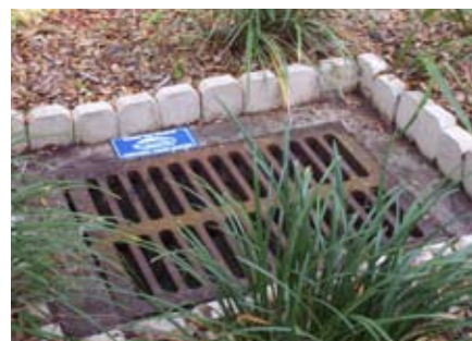
Figure 6.6: Existing storm drains
