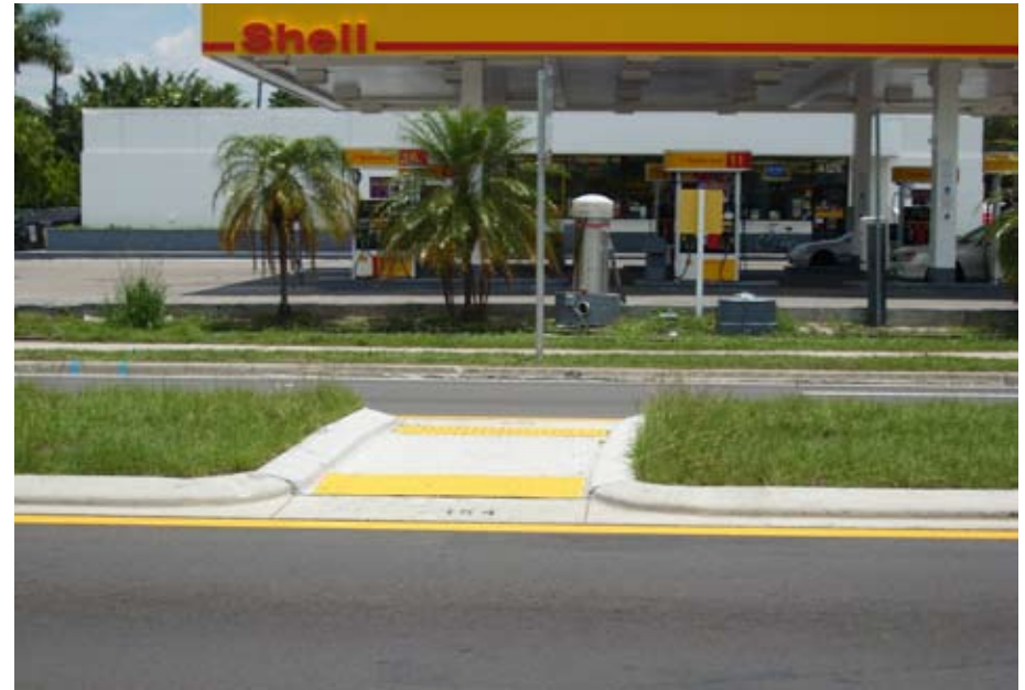
Figure 5.7: Median pedestrian crossing; opposite curb does not have a ramp for wheelchair access.
