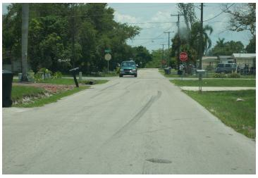
Figure 5.16: Typical Street on South Side of Palm Beach Boulevard, two 9' lanes, swales, no sidewalks.
