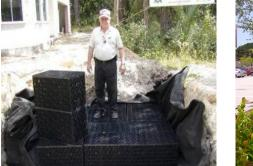
Figure 6.17: Exfiltration tank
