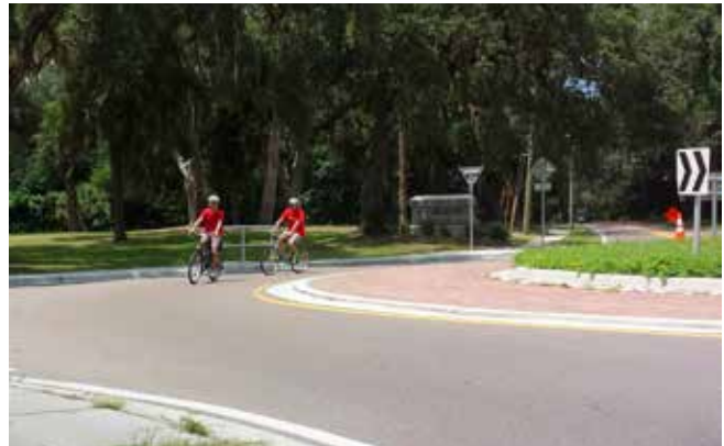
Roundabouts provide horizontal deflections. Location: First Coast Highway, Amelia City, FL Source: FDOT
