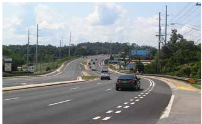
Narrower travel lanes help manage speed and provide for wider bike lanes. Location: Capital Circle NE, Tallahassee, FL Source: FDOT
