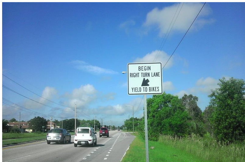
Bike lane markings at intersections with right-turn lanes (Credit: City of Fort Myers)
