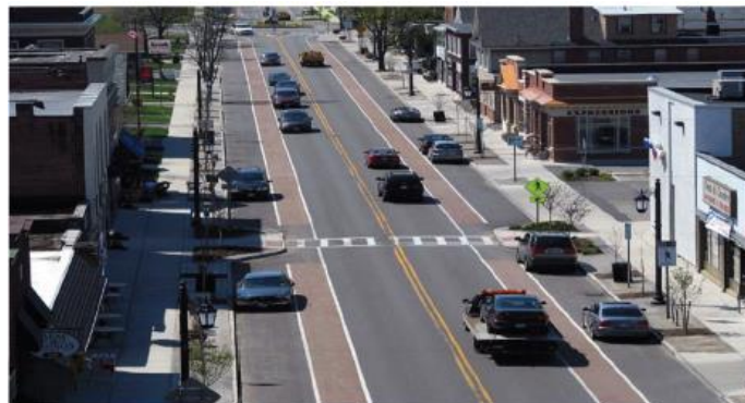
Parking assist lane (Credit: Michael Wallwork)
