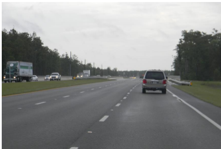
High automobile level of service, but poor multi-modal level of service (Credit: City of Fort Myers)
