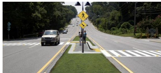
Staggered median crossing (Credit: Marcel Schmaedick)
