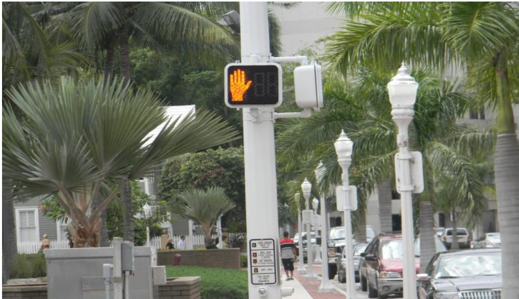
Sidewalks constructed adequate design guidelines (Credit: City of Fort Myers)
