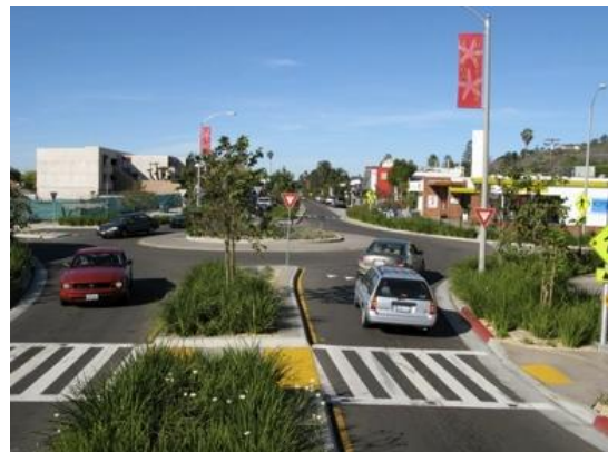
Roundabout: San Diego, CA (Credit: Michael Wallwork)
