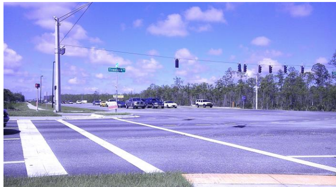
Controlled intersection (Credit: City of Fort Myers)
