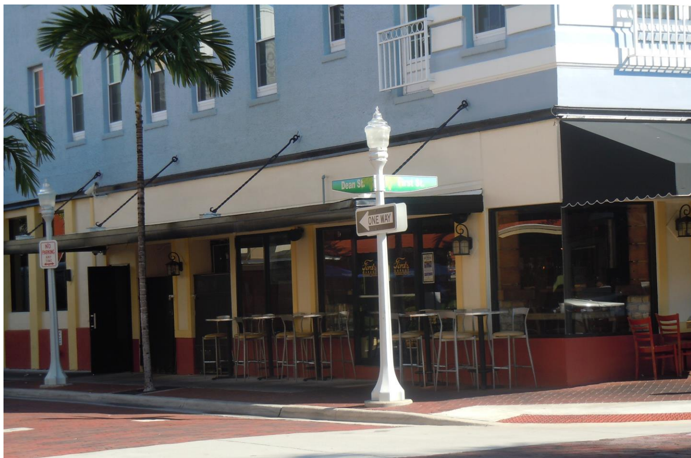
Dean Street- Street Lighting
