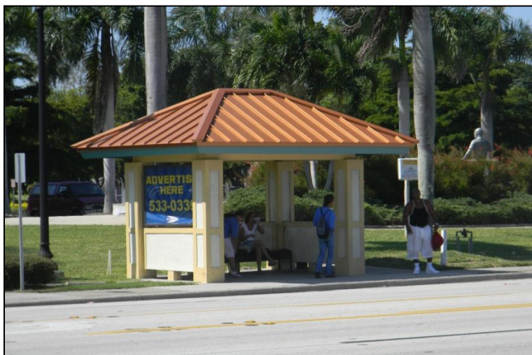
Comfortable public transportation stop (Credit: City of Fort Myers)
