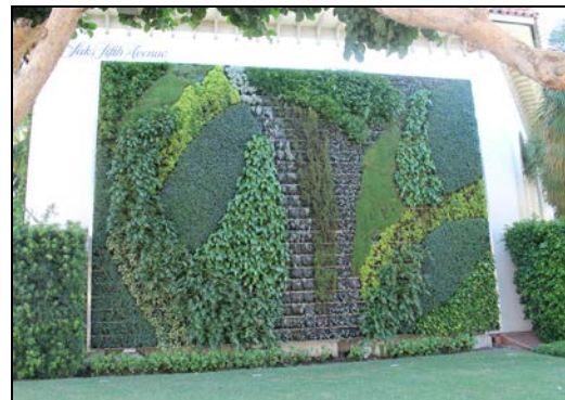
Figure 4.4.13-29 Character Example of Living Wall
