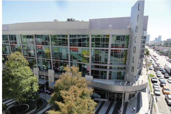
The Lincoln Theater has the building circulation located along the streets, behind an architectural glass façade, screening the large expanses of blank walls within the movie theater.
