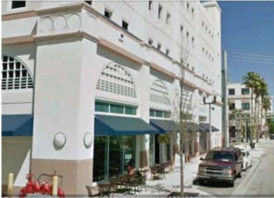
The Clematis Street garage utilizes consistent building materials with fenestration patterns to establish an attractive façade screening the parking levels over the retail space.
