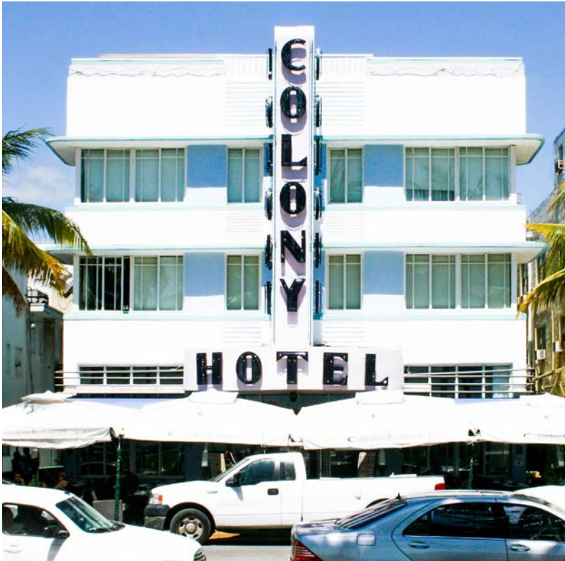
THE COLONY HOTEL, MIAMI BEACH, FL.. Architect: Henry Houser, 1935.
