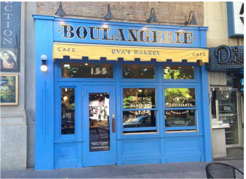
155 MAIN STREET SALT LAKE CITY, UTAH This storefront has a facade with a high base, framed openings, and traditional detailing. Though the overall facade transparency is lower using a taller base line, the location of the windows provide a clear view into the store for passersby.
