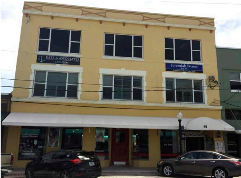
49 SW FLAGLER AVE. STUART, FL. A mixed use building with storefronts on the ground floor and an entry providing access to upper story offices. The facade is comprised of a three bays. Ornamentation is a simple cornice line between the first and second stories, an articulated parapet, and lintels over second story windows.
