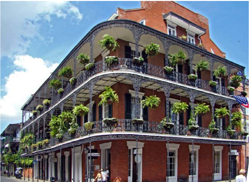
FRENCH QUARTER, NEW ORLEANS, LA. New Orleans was founded by the French, and occupied by the Spanish before being part of the Louisiana purchase. This eclectic style includes stacked porches, surrounding masonry structures, awnings, and expressive parapet and end walls.
