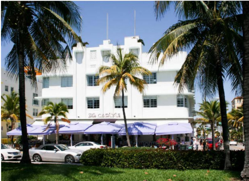
THE CARLYLE, MIAMI BEACH, FL. Nautical references are apparent in this Miami Beach hotel. Three centralized vertical piers stretch above the building's parapet and culminate with metal mast-like poles. The streamlined style, popular in the era, is evident in the rounded corners of the building, and the recessed ground floor.
