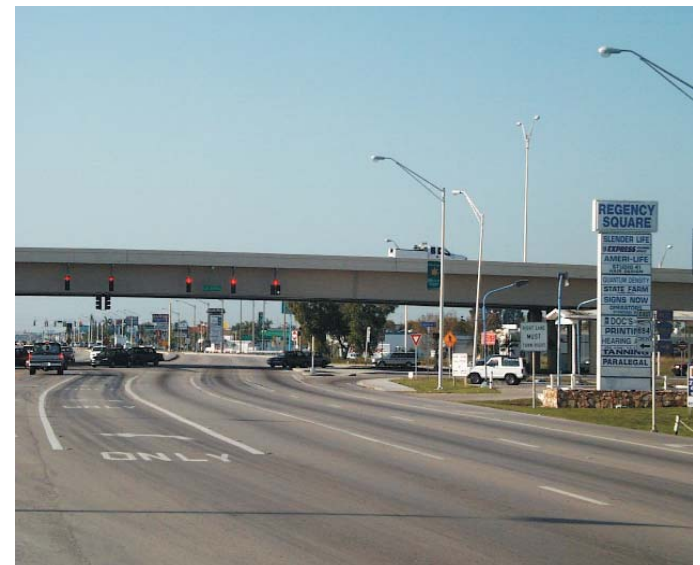
Grade-separated interchange in Lee County
