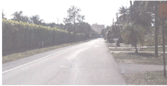
Figure (5) Bicycle / pedestrian access forbidden. No more physical barriers precluding access to adjacent land uses
