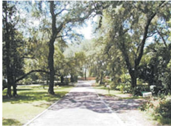
New rural road connections can be very narrow, with built-in traffic calming.
