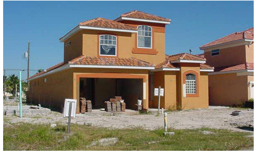
An example of a new home under construction in Naples Park
