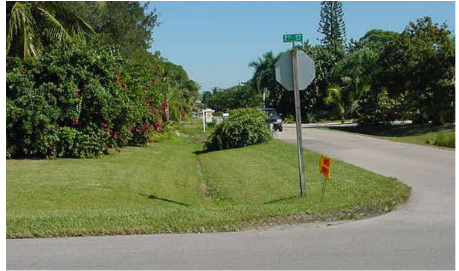
An open drainage swale
