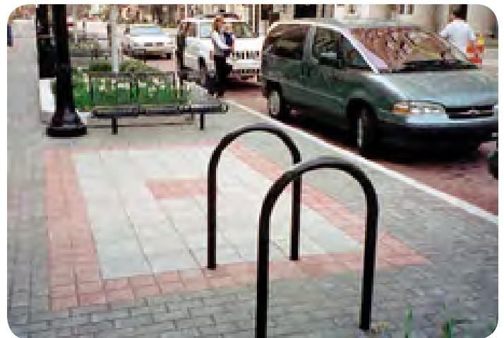
U-Racks Installed on a Sidewalk
