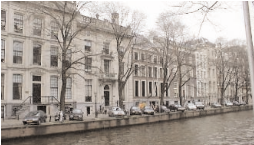
Rowhouses along the Herengracht, Netherlands
